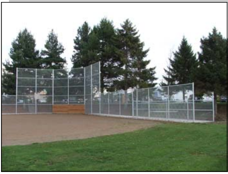
New backstop and wing fence at Soundview Field #4
